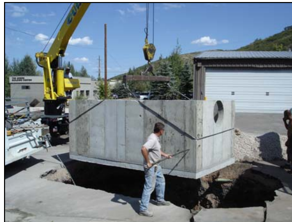
Picture 4: Public Works separator installation.
