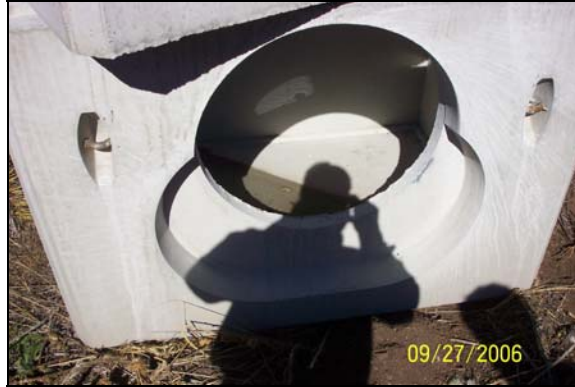
Picture 11: 8" Silt Trap.
