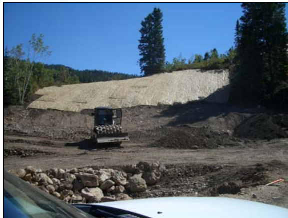
Picture 10: Alice Lode Steep Slope Stabilization.
