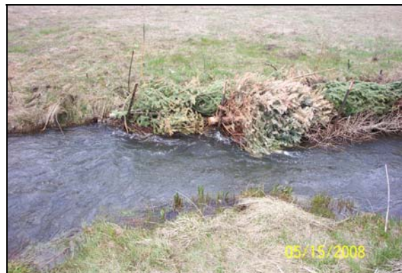
Picture 3: Weber Basin Job Corp Revetments.
