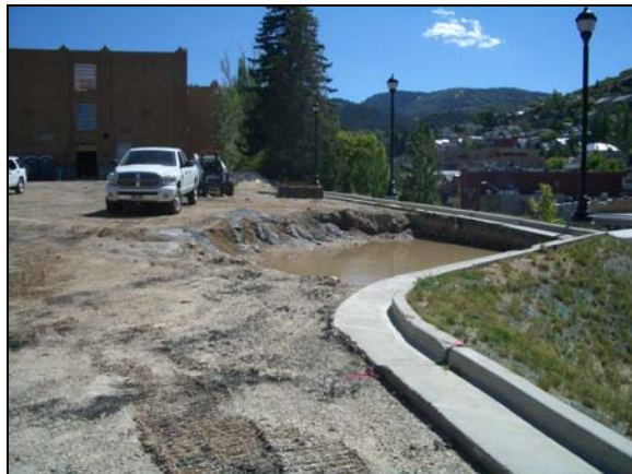
Picture 8: Detention Basins at City Hall renovation.
