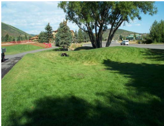
Picture 8: Golf Course Storm Water Settling Basin
