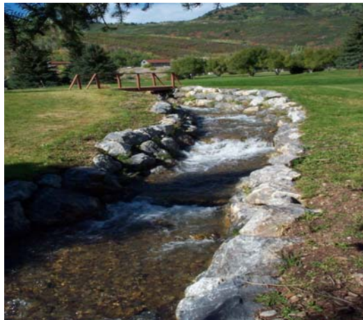
Picture 6: Hole 14 Stream Embankment Improvements
