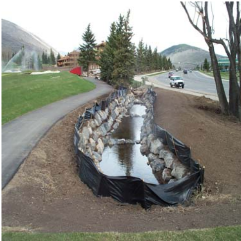
Picture 4: Park Ave outfall June.
