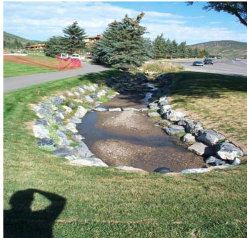
Picture 5: Park Avenue outfall September.
