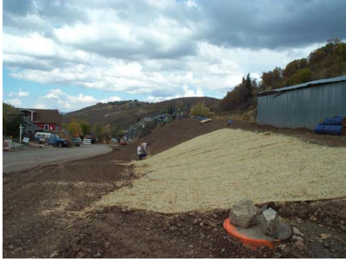
Picture 2: Installation of BMP – Marsac Sewer Project
